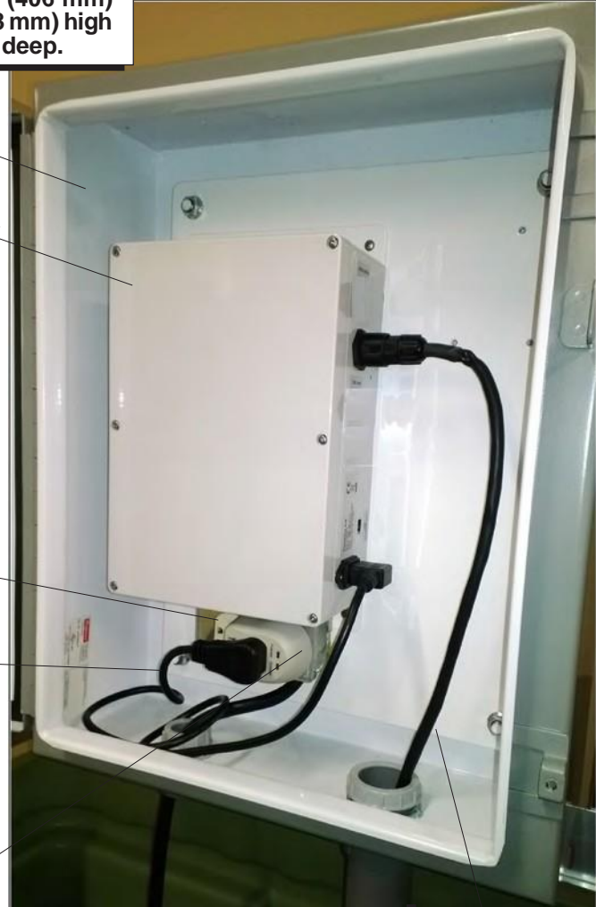
Integrated Power Supply Unit (IPSU)
