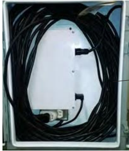
Coil Excess Cable Inside Electrical Box
